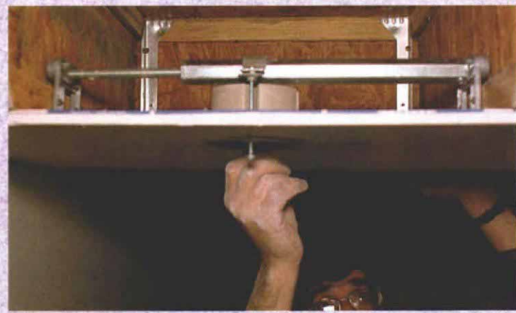
Specially designed ceiling box hangs from bracket.
