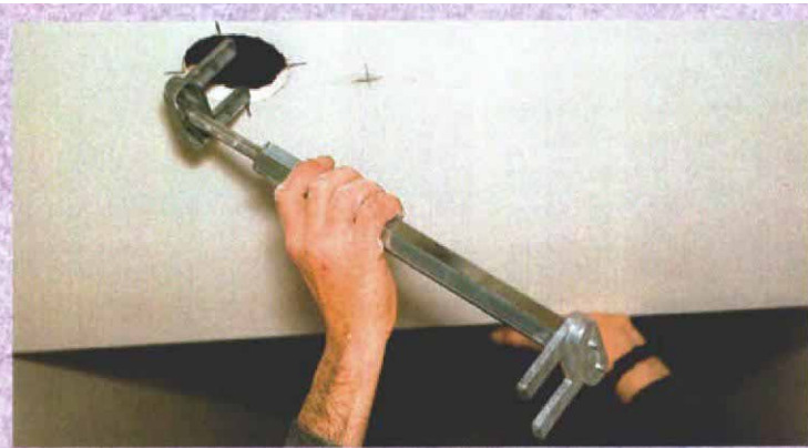
Remodeling bracket fits through a 4-in. hole.
